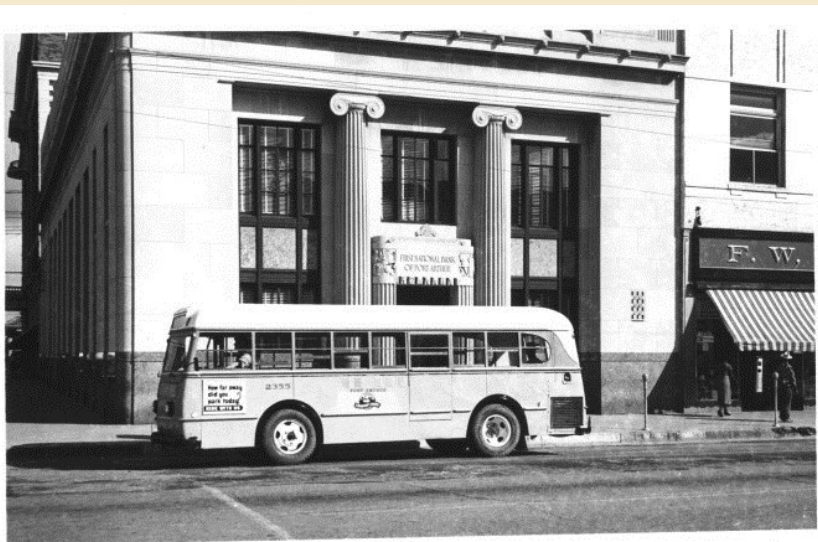
First National Bank Building in Port Arthur, Texas, with city bus passing in front
