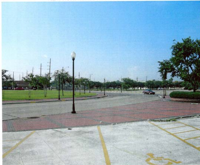
VIEW SOUTHERLY ALONG PEARL STREET CONNECTOR
