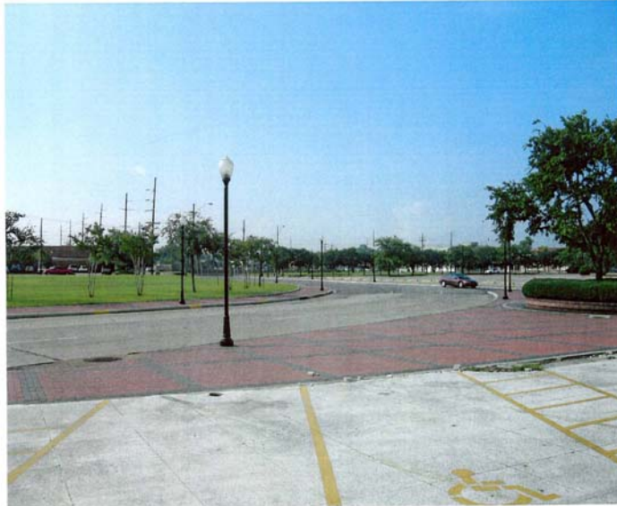
VIEW SOUTHERLY ALONG PEARL STREET CONNECTOR
