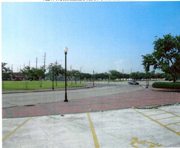
VIEW SOUTHERLY ALONG PEARL STREET CONNECTOR
