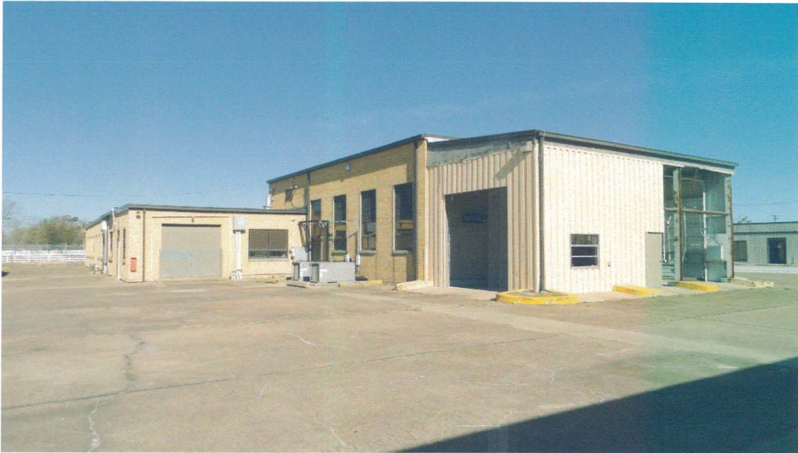
REAR & WESTERLY ELEVATION
