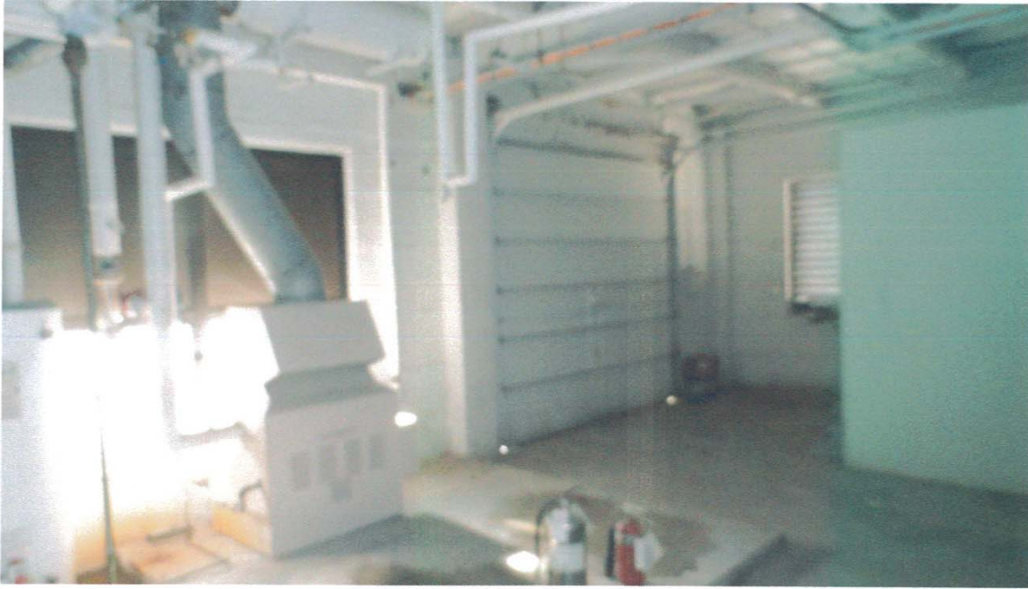
INTERIOR (Boiler room)
