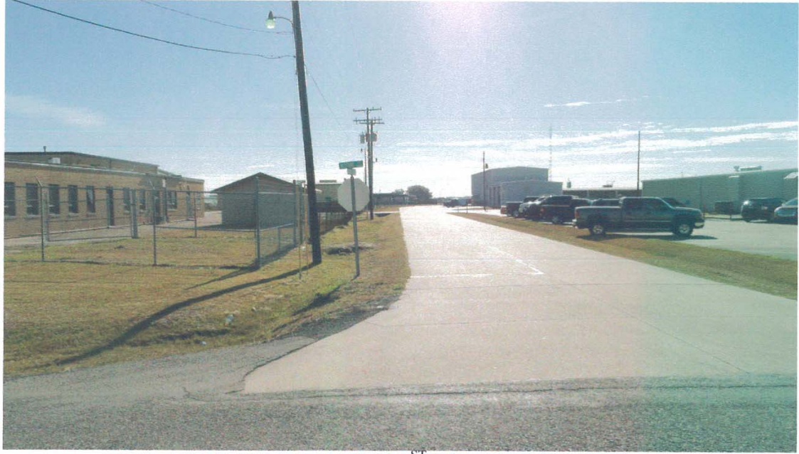
VIEW SOUTHERLY ALONG 1 ST STREET FROM VITERBO
