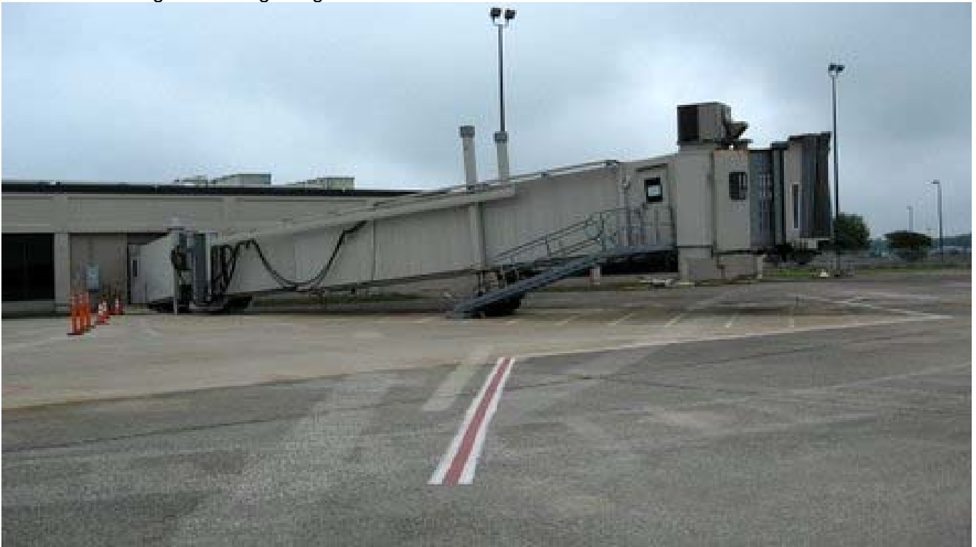
Photo of Passenger Boarding Bridge No. 2
