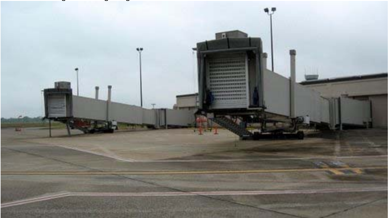
Photo of Passenger Boarding Bridges 1 & 2
