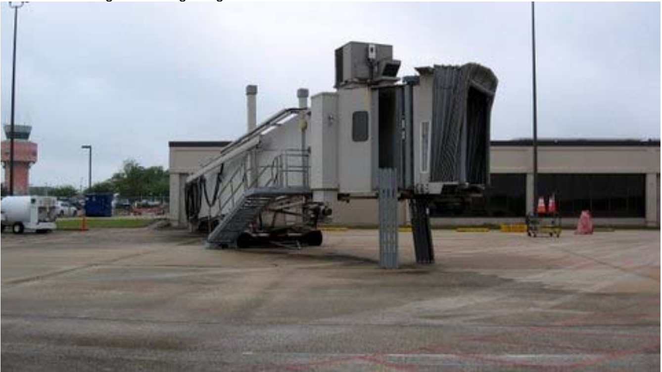
Photo of Passenger Boarding Bridge No. 1
