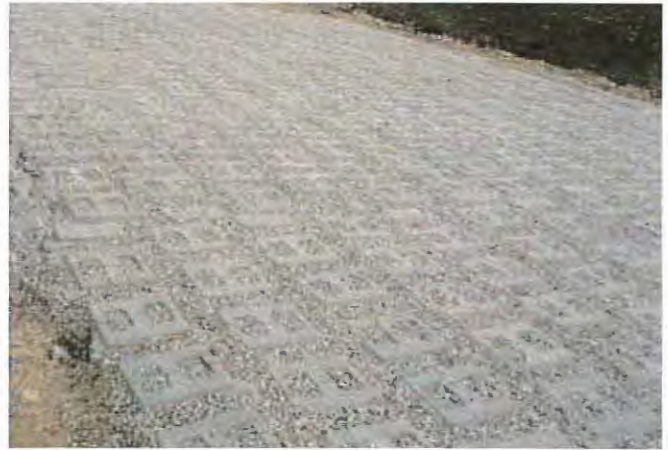
Backfilling should occur as early as possible to protect the filter fabric from UV damage.
