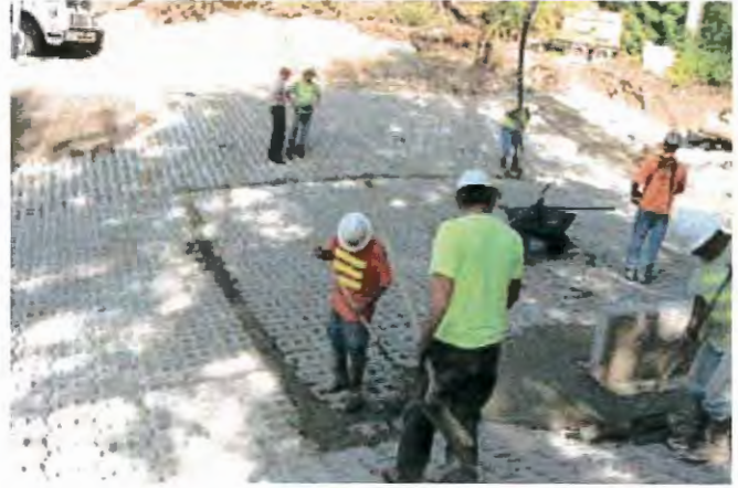
Grout to the top of the block or slightly lower — not above.
