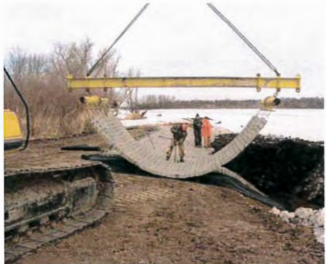
To assist in aligning the unit being placed, use of a pry bar may be necessary.
