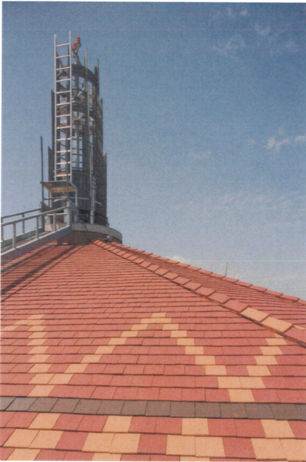
Multi-colored clay tile roof and restored spire, 2008.
