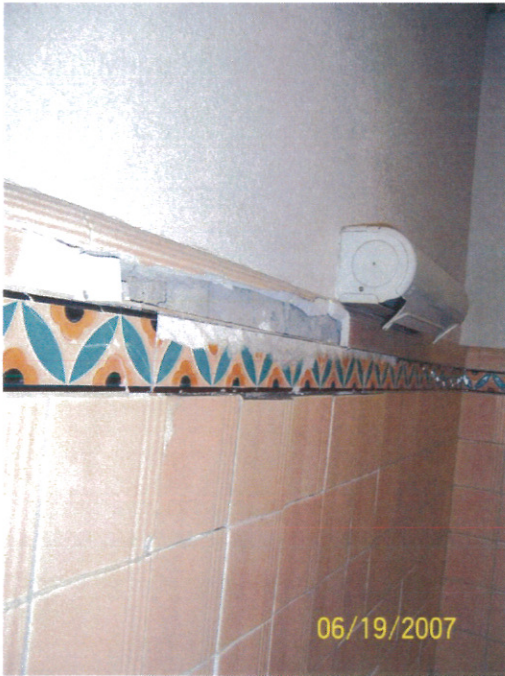
After Masonry Restoration Ph. 3 023-03 Restroom tile damage
