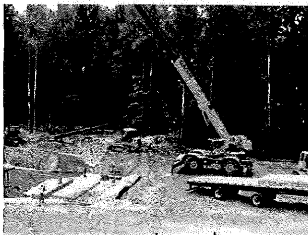
The use of a crane is optimal for fast and safe unloading and installation of the mats.
