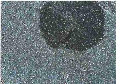
Deficiency: There are punctures, cracks or splits in the roofing membrane which allows water into the roof system and/or building.
