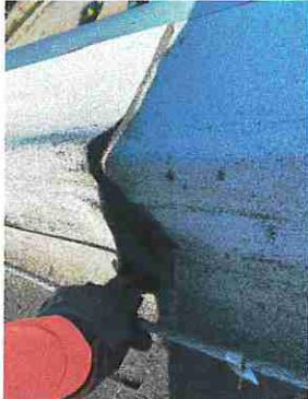
Deficiency: The existing base flashing have failed and are in need of replacement.
