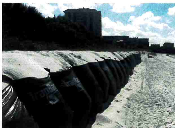
Exhibit 8. Trap Bag Installation in Volusia County, Florida
