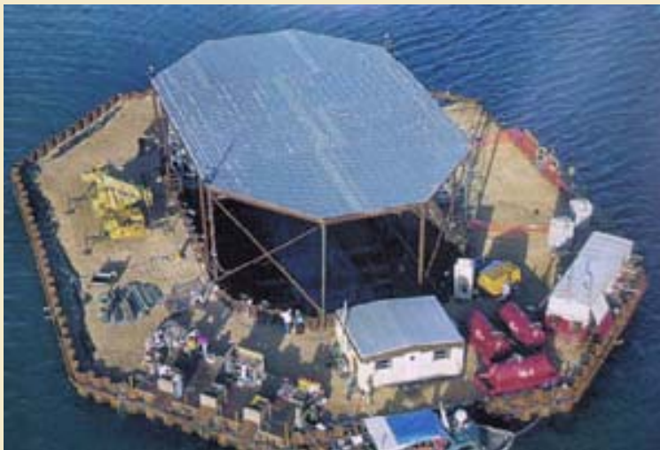
Images of the cofferdam built for the excavation of the ship La Belle in Matagorda Bay, Texas, and the first of 3 bronze 4-pounder cannons discovered in the hold of the ship.
