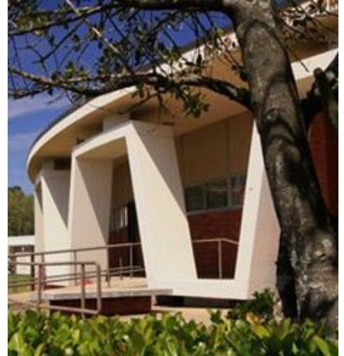
Otho Plummer Administration Building Photo Credit: Lamar University website
